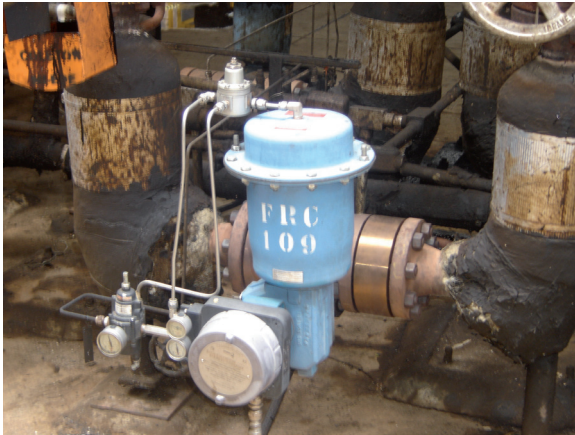
Figure 2: Eccentric rotary plug valve, Neles Finetrol™, provide reliable, long-lasting performance for heater pass control.
